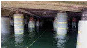
Ángel Franco/The New York Times Piers ready for a cement pour.
