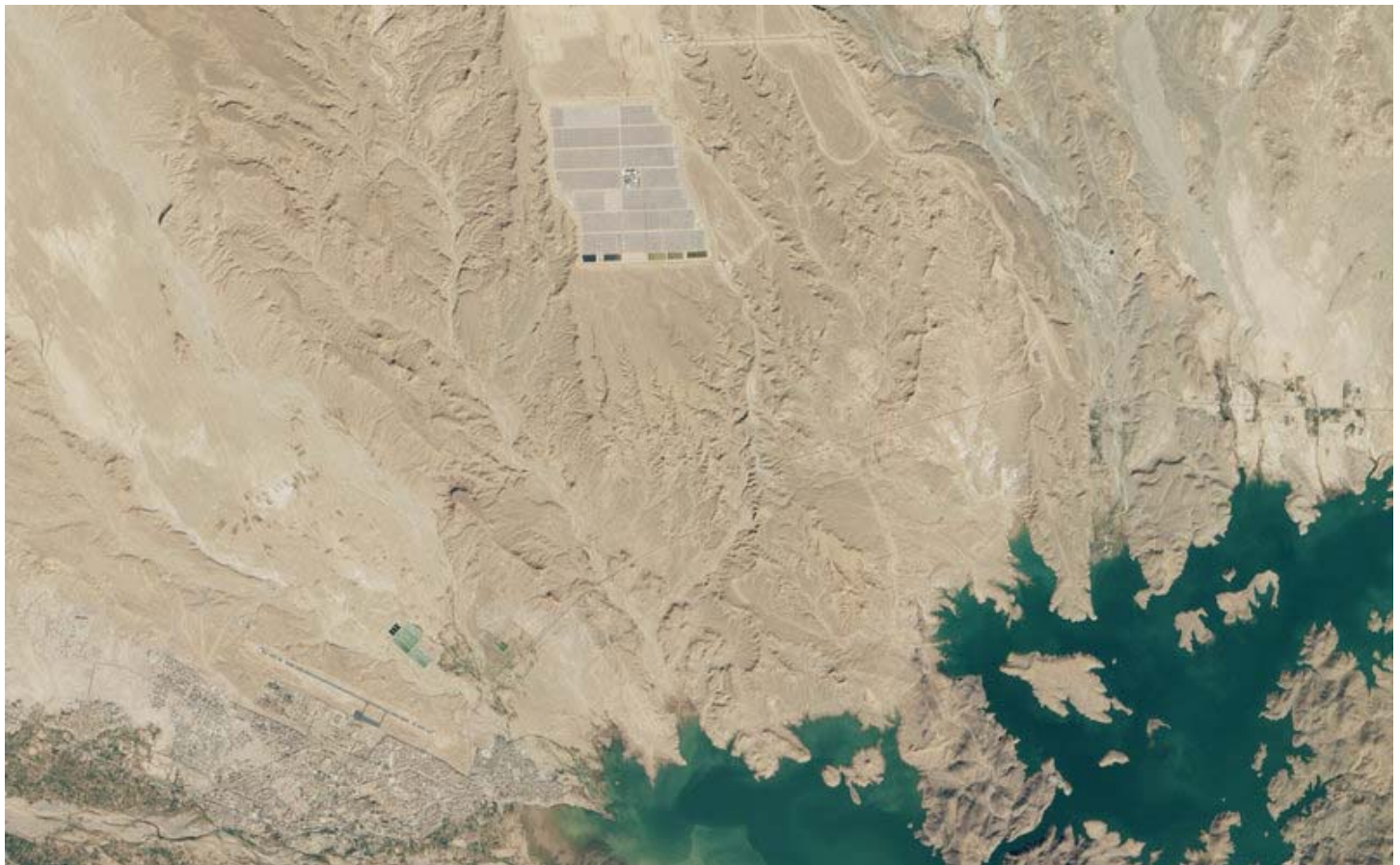
The Noor I power plant as seen from space. In the lower left, you can see the Moroccan town of Ouarzazate; in the lower right is the reservoir that is supplying the plant with water.
